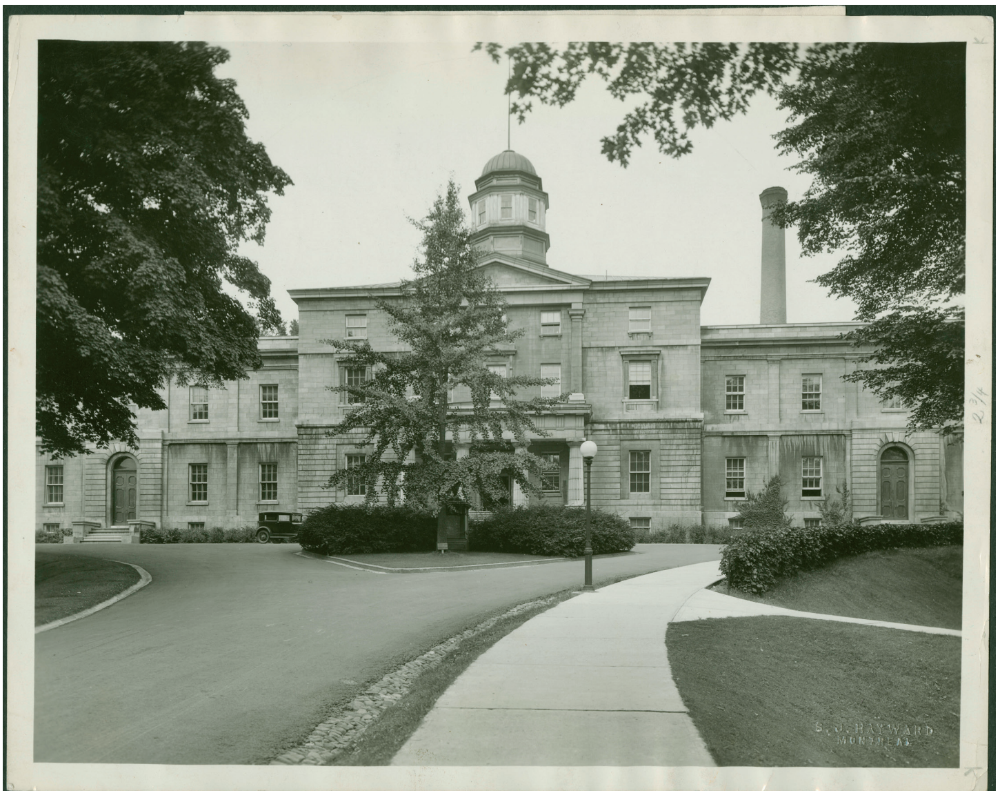
Figure 3. Arts Building, 1929, photographer S.J. Hayward, MUA PR026608
