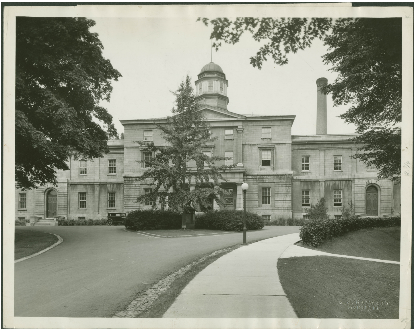
Figure 3. Arts Building, 1929, photographer S.J. Hayward, MUA PR026608
