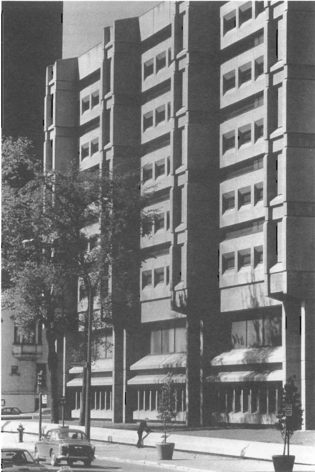
McLennan Library Building, ca. 1970. (McGill University Archives)
