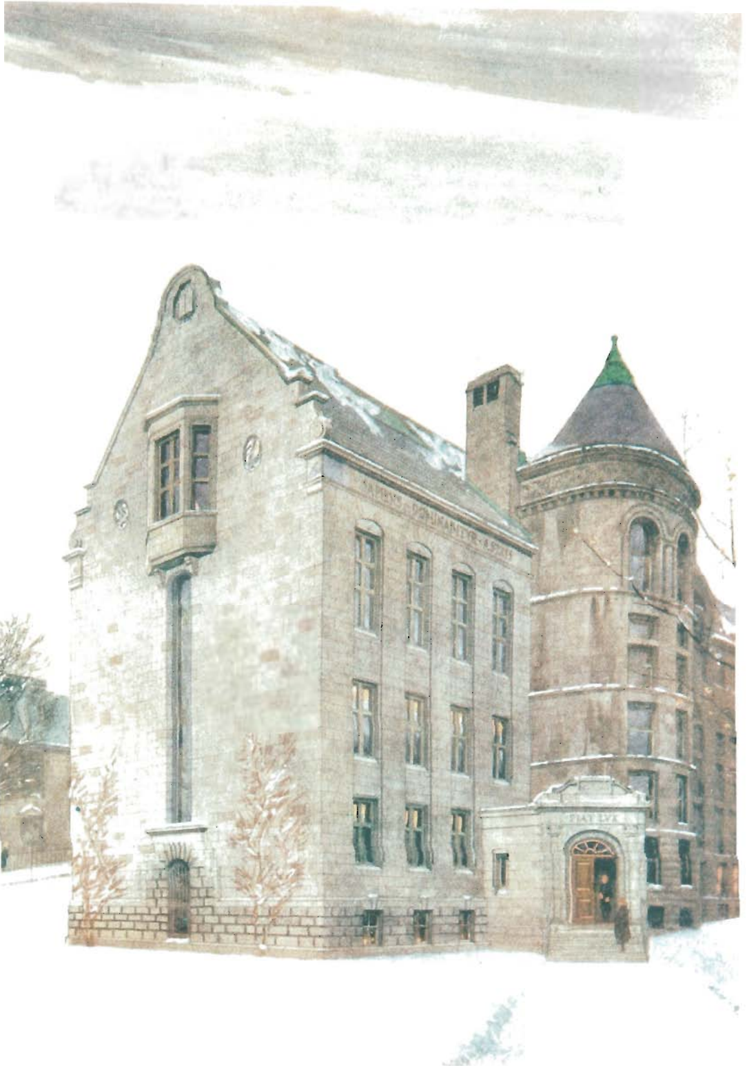
The 1921 addition by Percy Nobbs to the Redpath Library. ( Old McGill , 1923)
